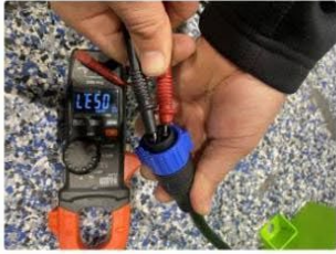
Voltage check for M8-Plug
