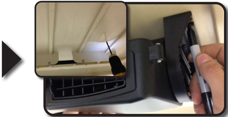
Insert the four 6mm x 45mm bolts through the top of the roof with rubber side of washer down as shown. If you are installing the fan on a TXT the four 6mm x 70mm bolts are needed.
