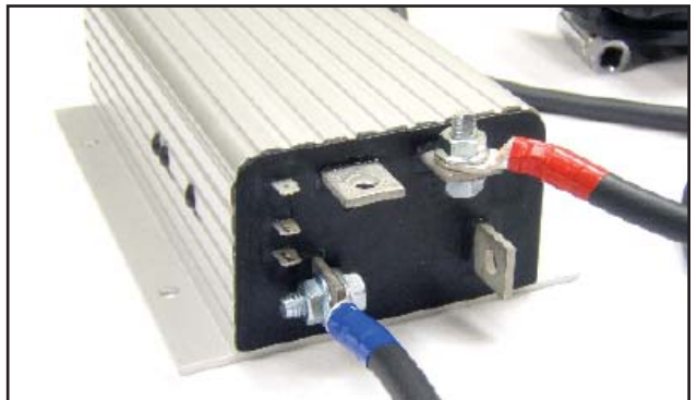
11f. Blue Cable Installation on Controller
