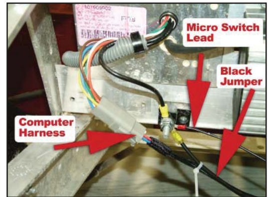
20. Install Computer Harness & Black Jumper
