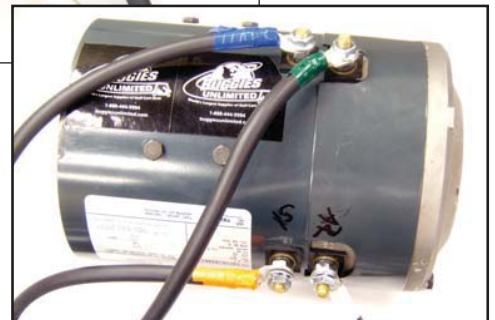
13g. Orange Cable Installation
